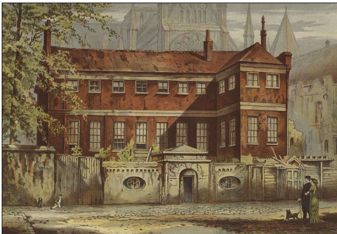
Ashburnham House, Old London, previous site of the Cotton Library. This collection of manuscripts was amassed by the antiquarian and bibliophile Sir Robert Bruce Cotton (1571-1631). In 1731 the collection was badly damaged by a fire in which 13 manuscripts were completely destroyed and some 200 seriously damaged. The most important Anglo-Saxon manuscripts had already been copied; the original text of 'The Battle of Maldon' was completely lost.
